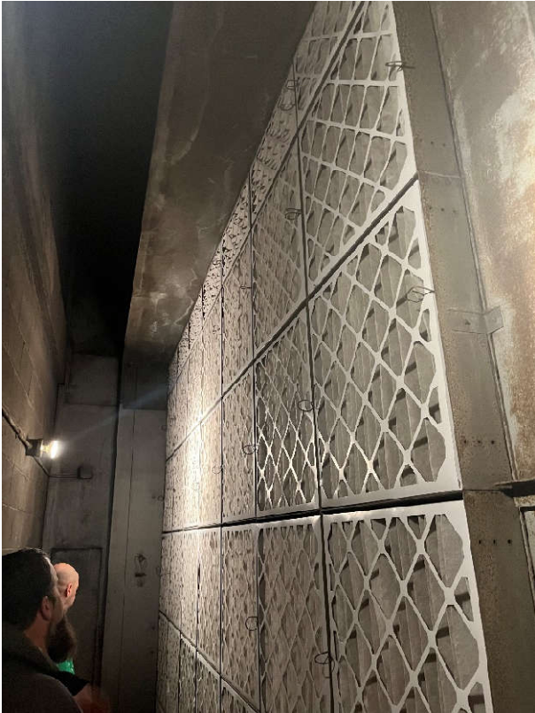
Typical Interior AHU Filter Wall
