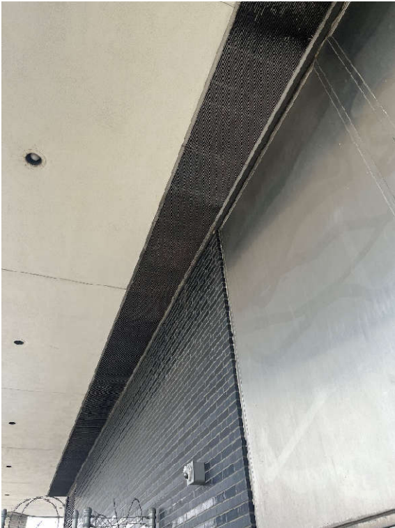
Typical (2) Overhang Intake Louver
