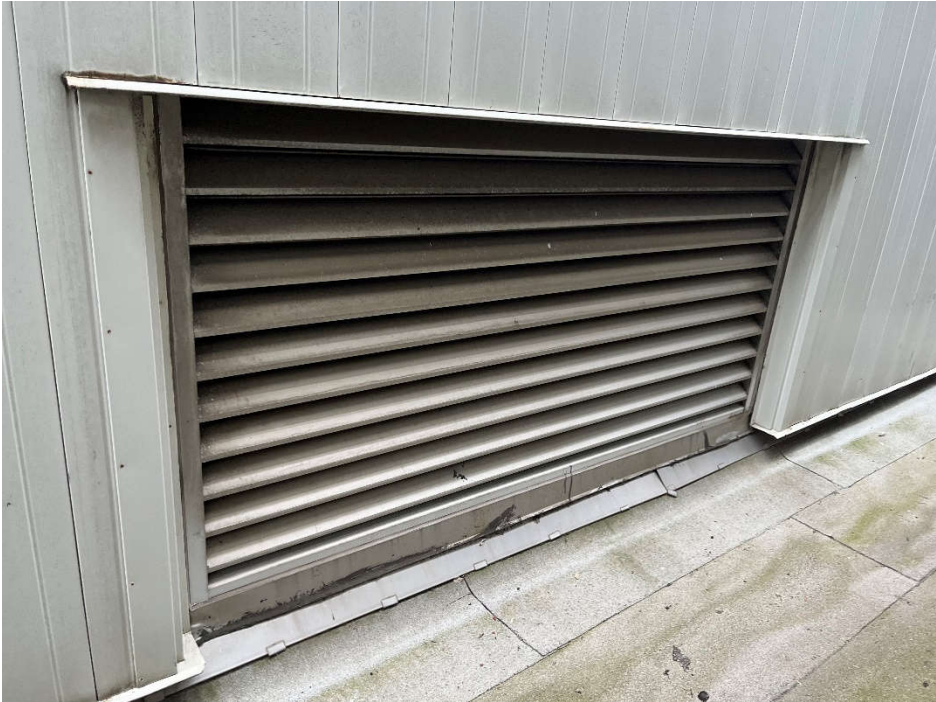
Typical AHU Outside Air Intake At Roof Level
