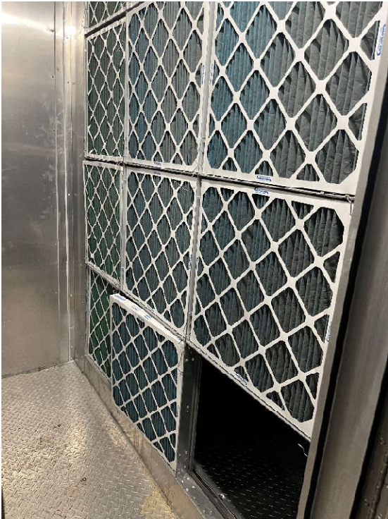
Typical (4) AHU Filter Section
