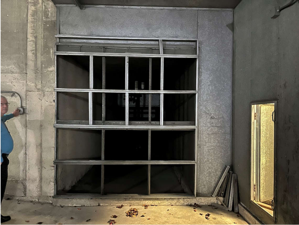
Typical AHU Outside Air Intake damper (Inside of AHU)
