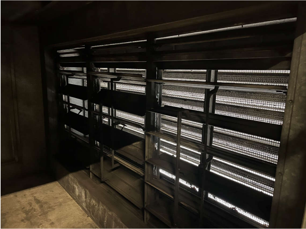
Typical AHU Outside Air Intake damper (Inside of AHU)
